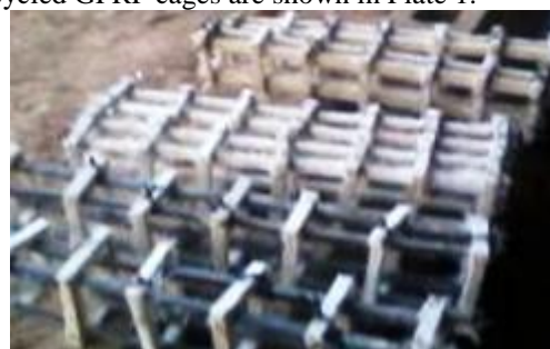
PLATE 1: Sample recycled GFRP reinforcement cages
